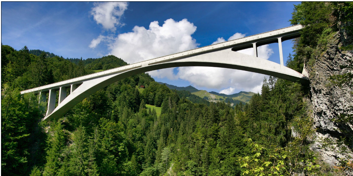
Figure 1 The Salginatobel bridge in Switzerland was designed by Robert Maillart, who formed the arch according to thrust line patterns (Rama 2008)
