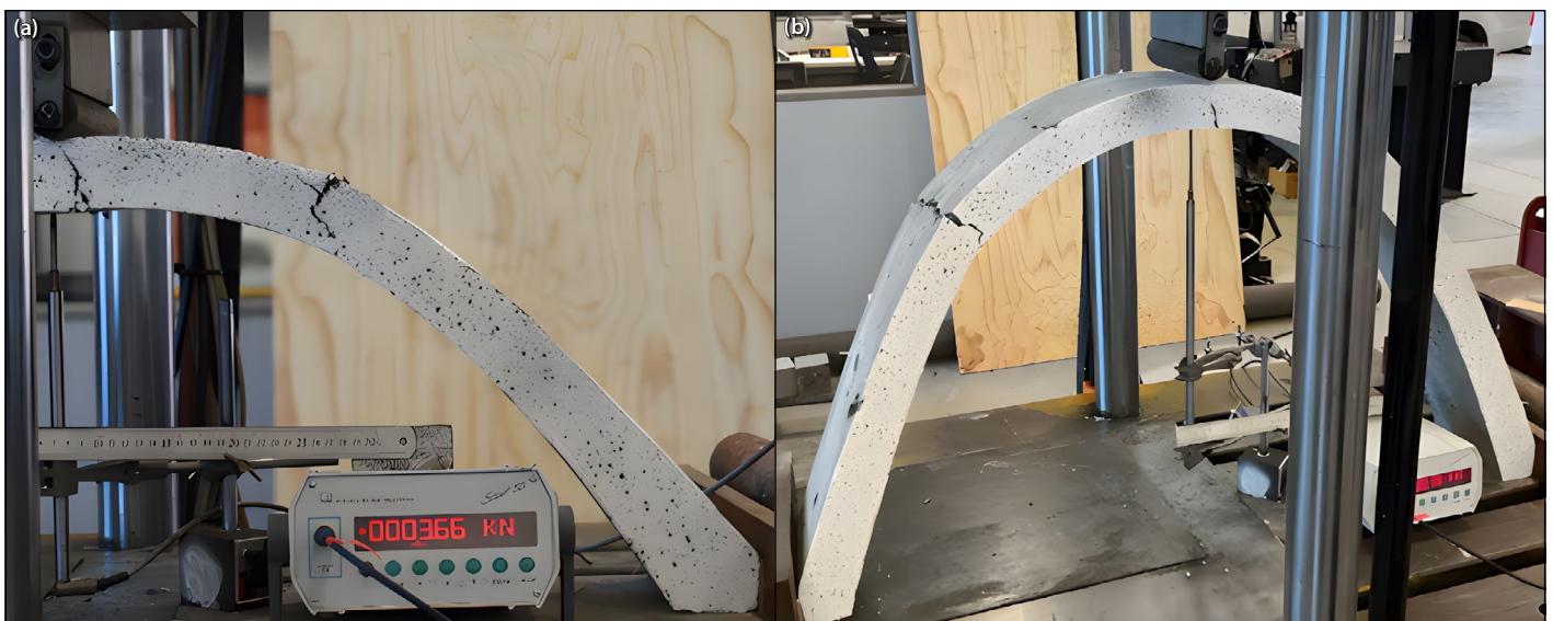
Figure 18 Both the shallow arch (a) and steep arch (b) formed a five-hinge failure mechanism
